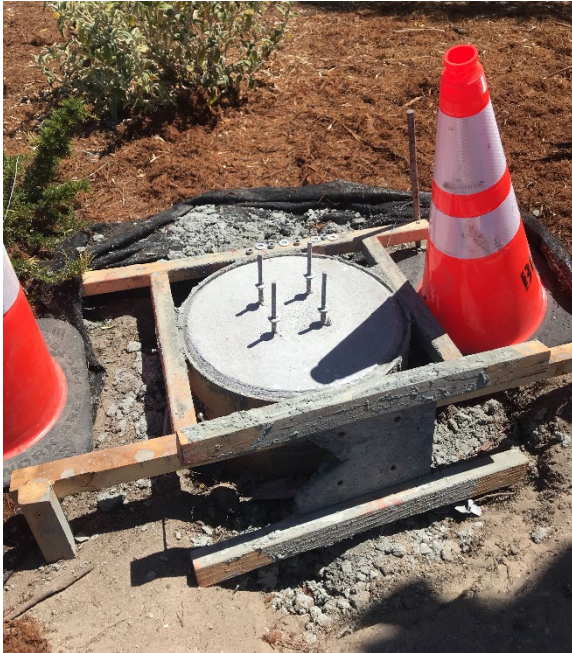
Wayfinding sign foundation construction
