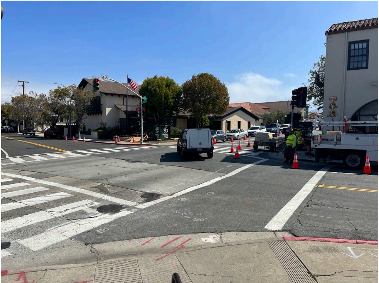
During Construction on Munras Avenue at Webster Street, 2022
