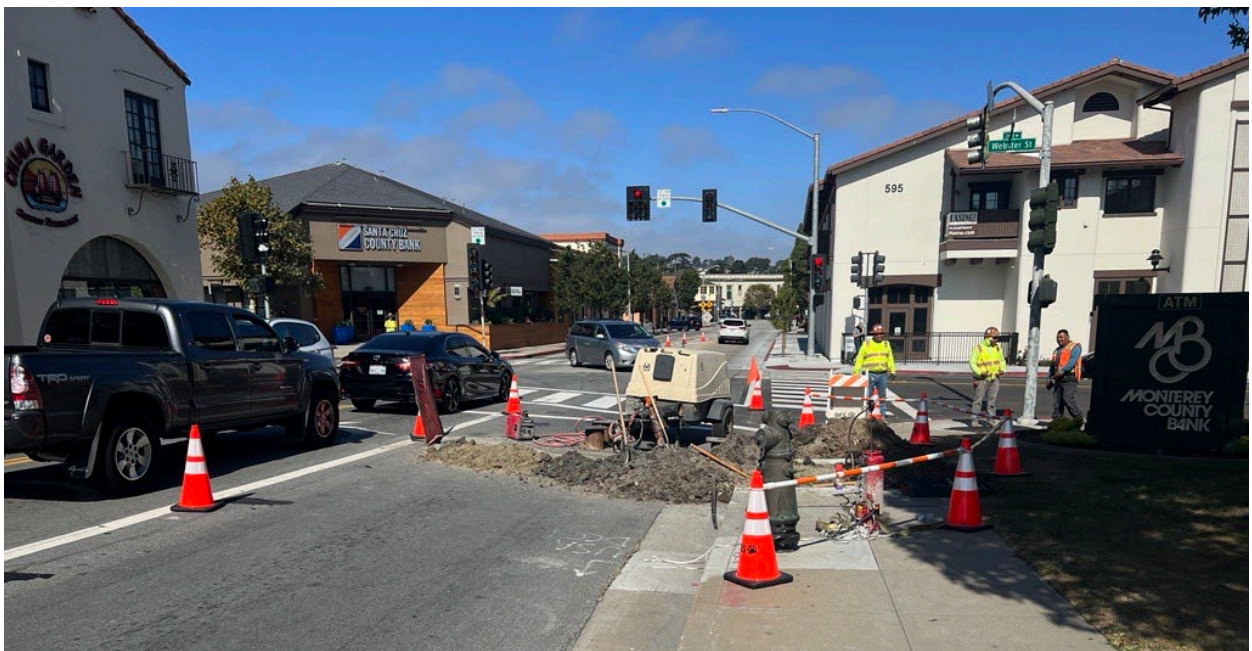
During Construction on Munras Avenue at Webster Street, 2022
