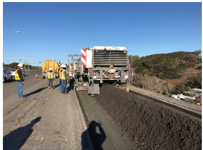
Recycled of pavement grindings
