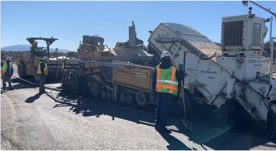
Rear of CIR Train – Paving Machine & Roller
