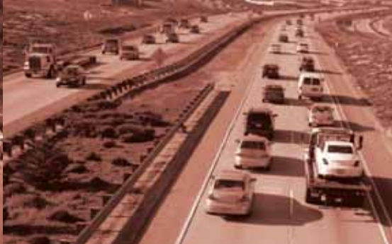
Widening of Highway 1 in Seaside/Sand City
