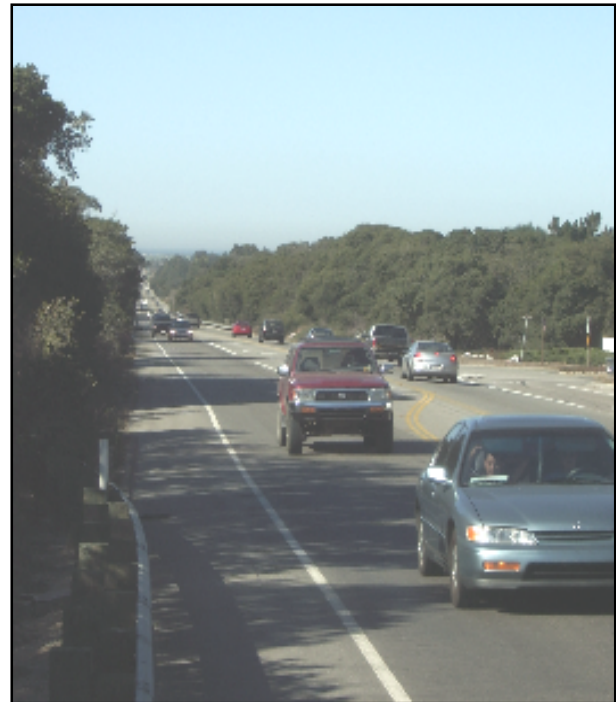
Looking westbound on SR 156
