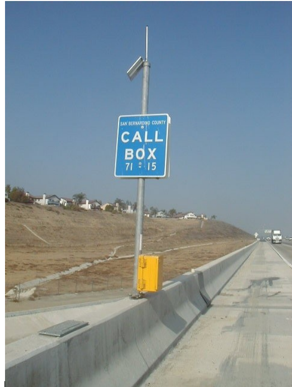
Site Type H or K – installed on a k-rail or concrete barrier.
