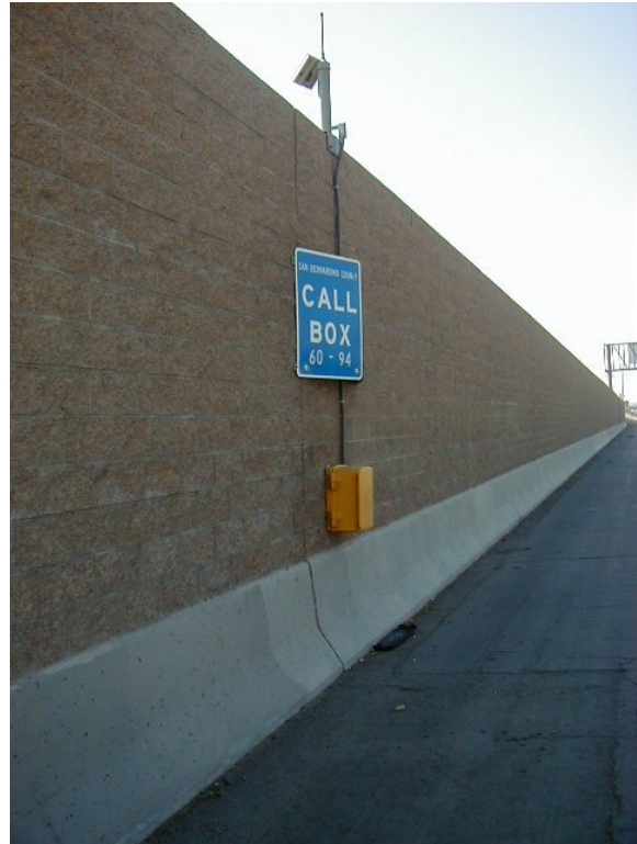
Site Type D – mounted on a soundwall.
