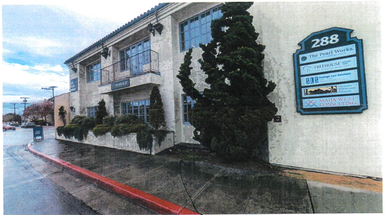
LEFT SIDE OF BUILDING
