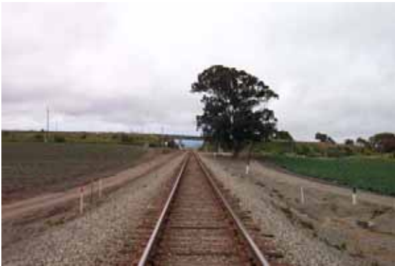
Castroville Station Location, South View
