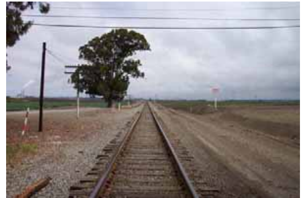
Castroville Station Location, North View
