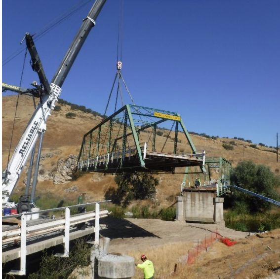
Demo of existing bridge
