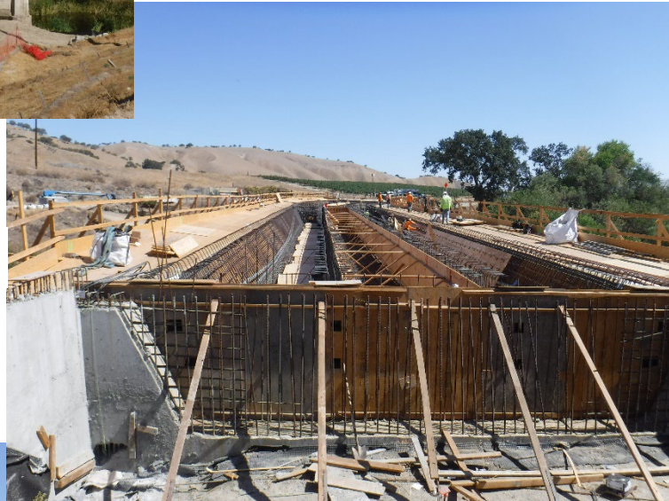
Box girder construction
