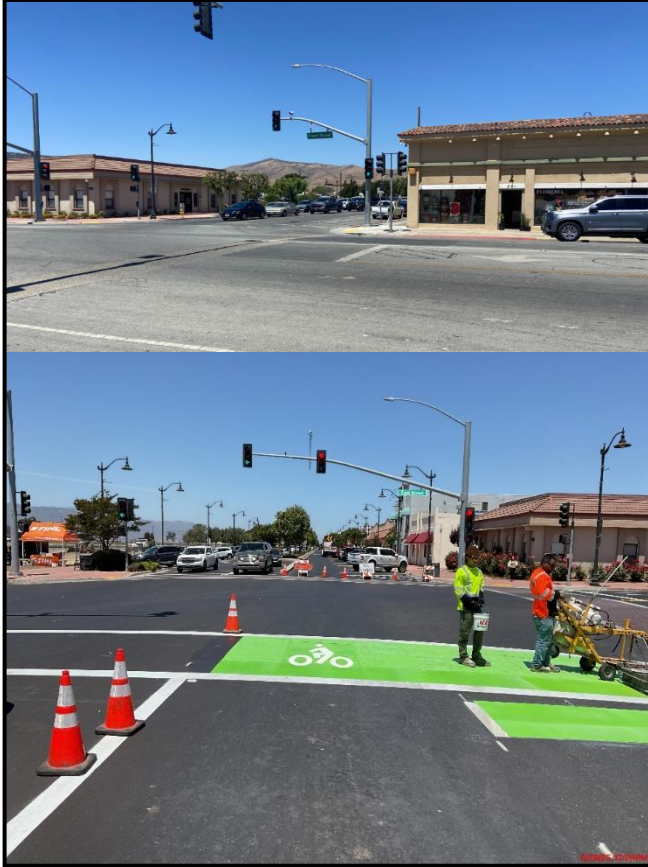
Figure 3 - Enhanced Striping Improvements on Newly Paved Streets (Front at East St) Before and After
