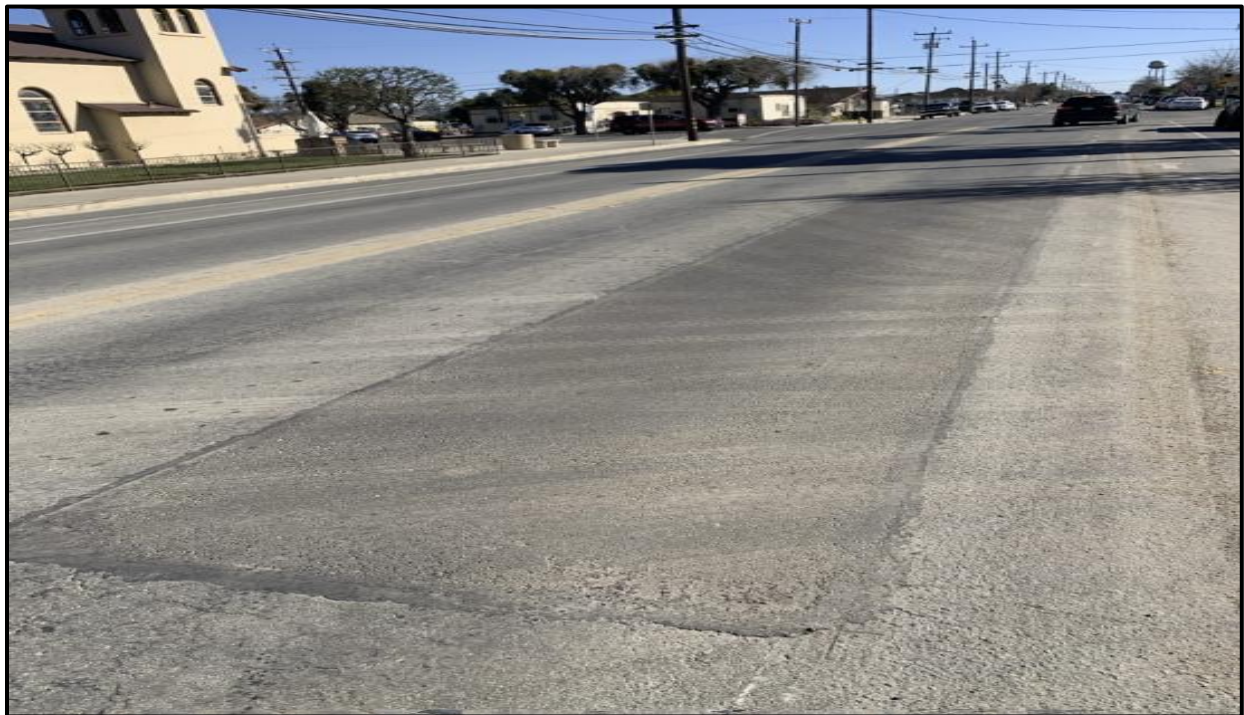
Figure 10 - Monterey Street Repair After Picture
