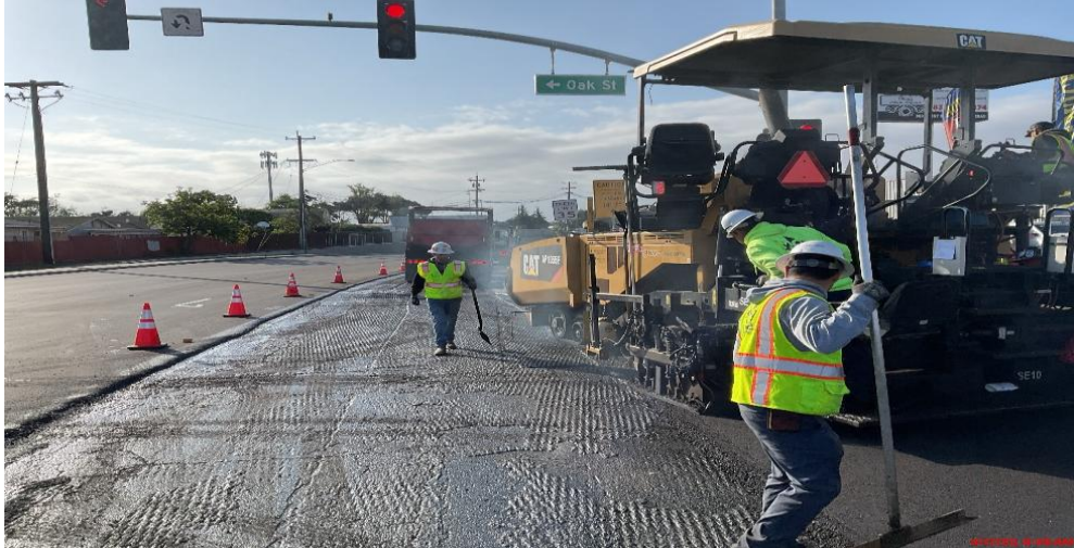
Figure 5 - Paving Operations on Front Street
