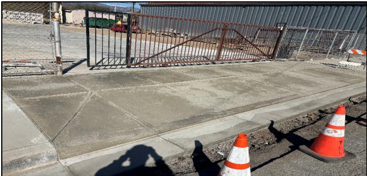
Figure 8 - State Street Sidewalk Repairs After Picture
