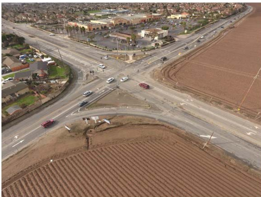
Existing Natividad/Boronda Intersection
