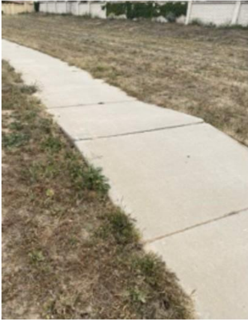
Figure 2 - Before: San Vicente Rd Repairs
