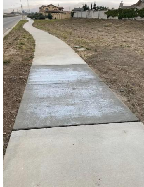
Figure 3 - After: San Vicente Rd Repairs
