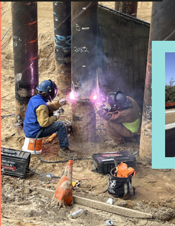
Welding sections of bridge piles together - FORTAG
