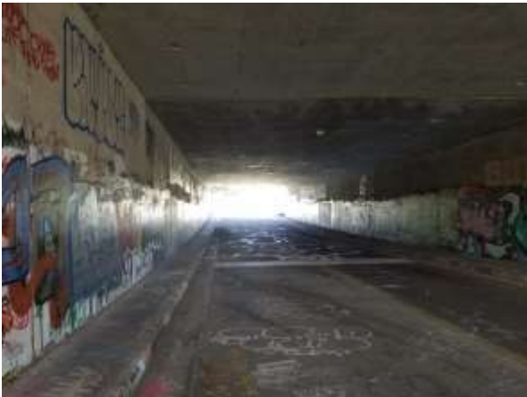
Photograph 10. CSUMB Loop South Segment - View of the bridge on the western portion of the Segment.
