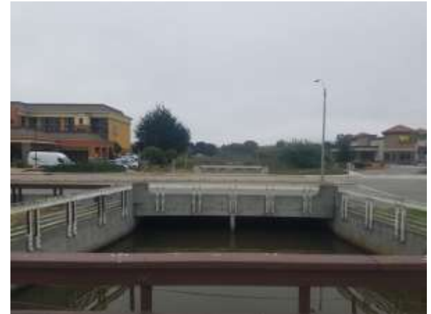
Photograph 15. Canyon Del Rey/SR 218 Segment - View of the lagoon and nearby properties on the western portion of the Segment, facing southeast.
