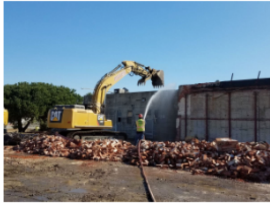
Demolition of 52 W. Market Street.
