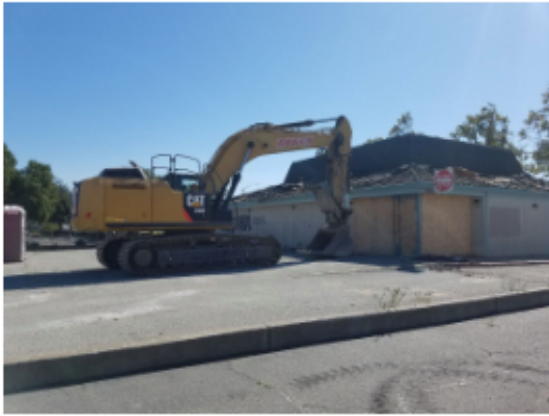
Demolition of the former Credit Union, located at 20 W. Market Street.
