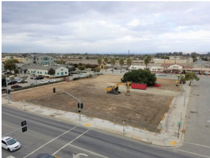
Structure demolition is complete.
