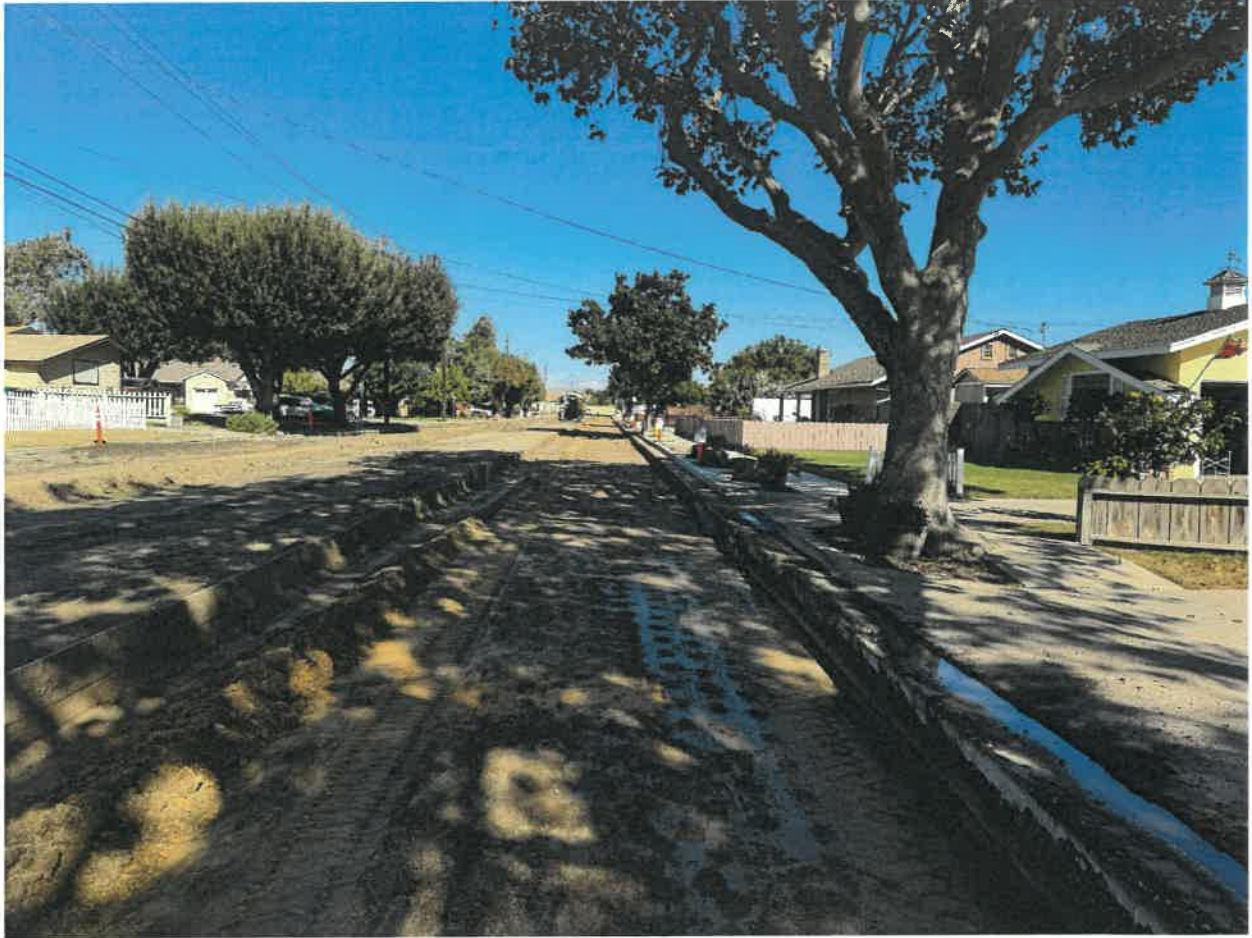
Figure 1 Division Street - During Construction
