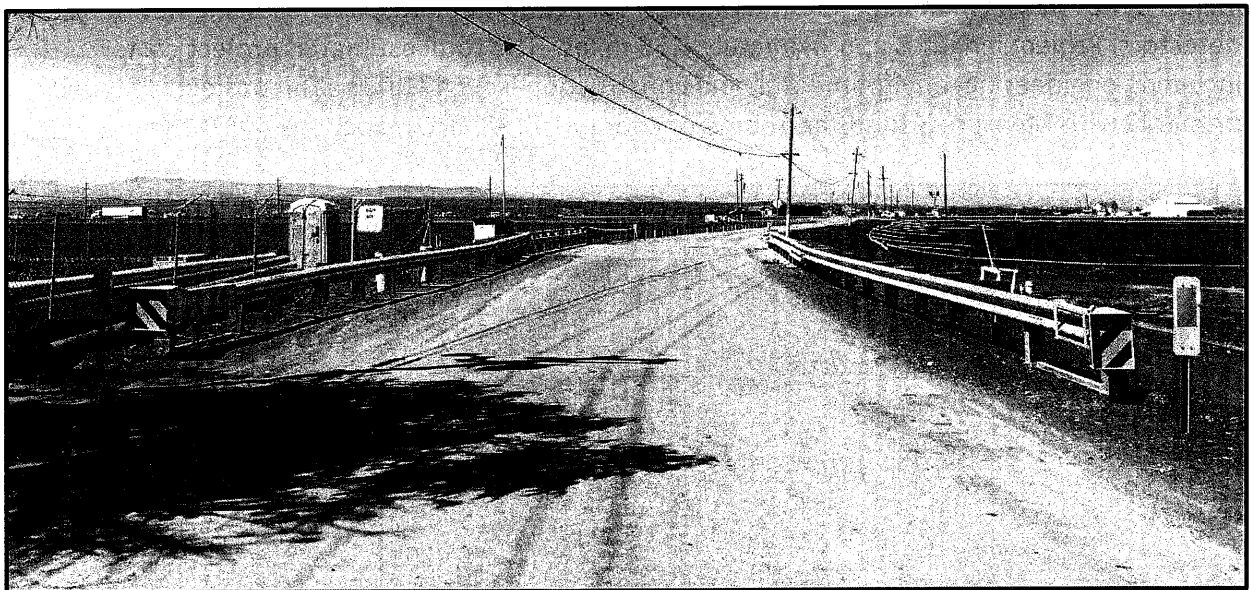
San Jon Road new bridge railing
