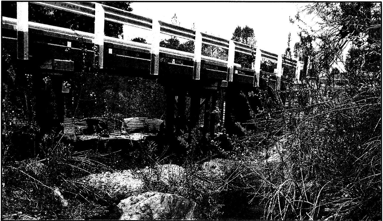
Old Peach Tree Road Bridge
