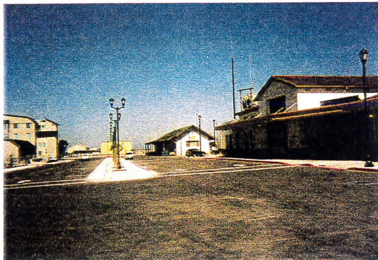
Station Building and Access Road
