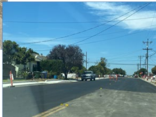
After, taken at the same location from the opposite direction (Drainage issues resolved, Note conformance curb, Driveway detail, wheelchair in the distance)
