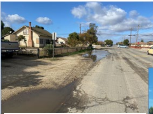
Before (Drainage issues, No sidewalk)
