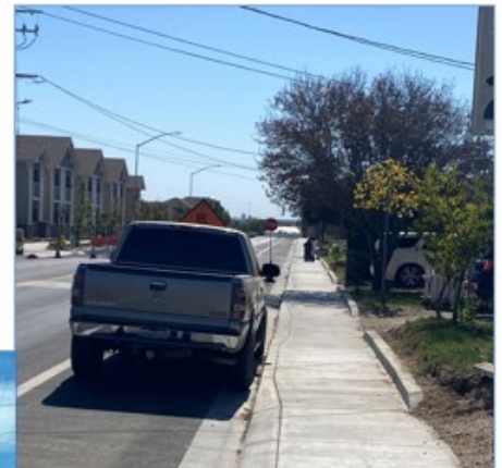
After, taken at the same location from the opposite direction (Drainage issues resolved, Note conformance curb, Driveway detail, wheelchair in the distance)
