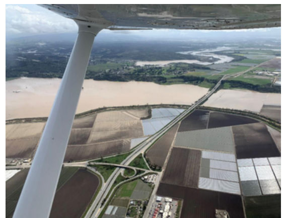
Aerial view of Highway 1 with the junction of Highway 129 in the foreground. The Pajaro River is mid-picture, levee breach can be seen in the background. Photo credit: Caltrans
