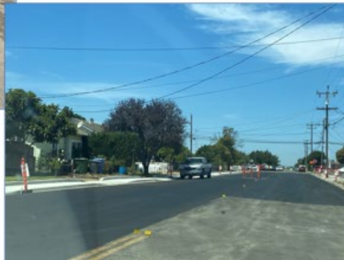
After (Drainage Issues resolved, New Sidewalk)
