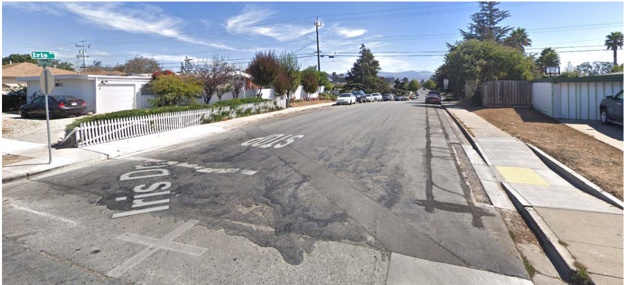
Tyler St. & Iris Dr. (during construction) with 2 ADA compliant ramps
