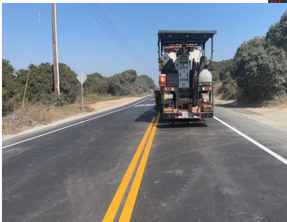
Placing Pavement Traffic Stripes
