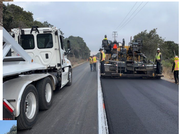
Placing Asphalt Concrete
