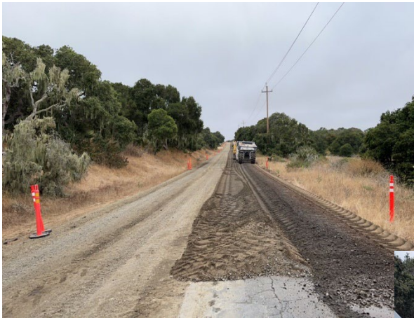
Full-depth reclamation process
