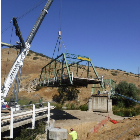
Demo of existing bridge
