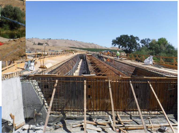
Box girder construction
