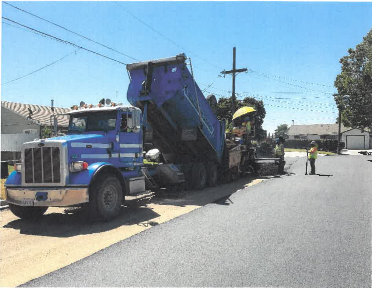
Figure 2 Repaving Vivian Drive
